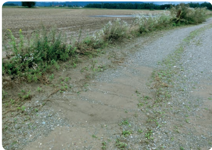
.... may lead to erosion even on flat surfaces.
